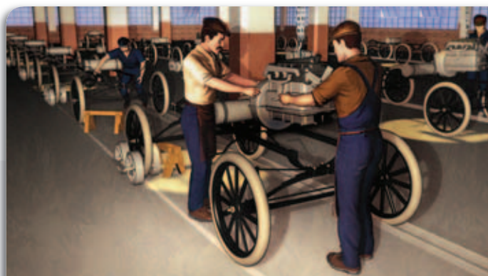
The chassis, or frame, and the engine are assembled on separate lines. Workers on a third line then attach them.
