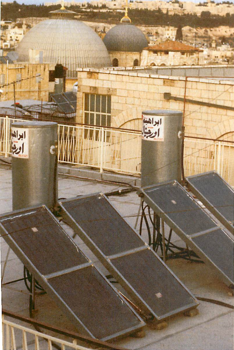
▲ FIGURE 9-48 SOLAR PANELS Solar panels installed on apartment rooftops in the Old City of Jerusalem are used to heat water, which is stored in the adjacent tanks. The domes are the Church of the Holy Sepulchre, built at the site where Jesus is thought to have been crucified, buried, and resurrected (see Chapter 6).
